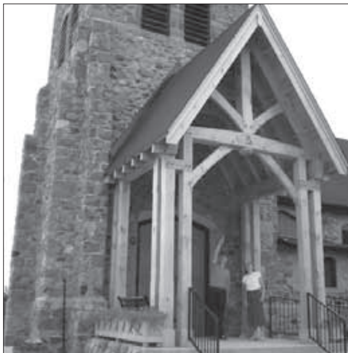
Above: The new covered porch on the South side of the Perrytown Anglican Church. This is a case of life imitating art. To make a set for the movie "Closing the Circle" a porch was "built" on to the church. The congregation so liked the fake movie porch that a properly constructed porch was added. On the inside there is a "stairway to Heaven" carved into the structure.
